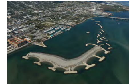
New Island Construction
