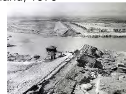
Banqiao dam failure; China, 1975
